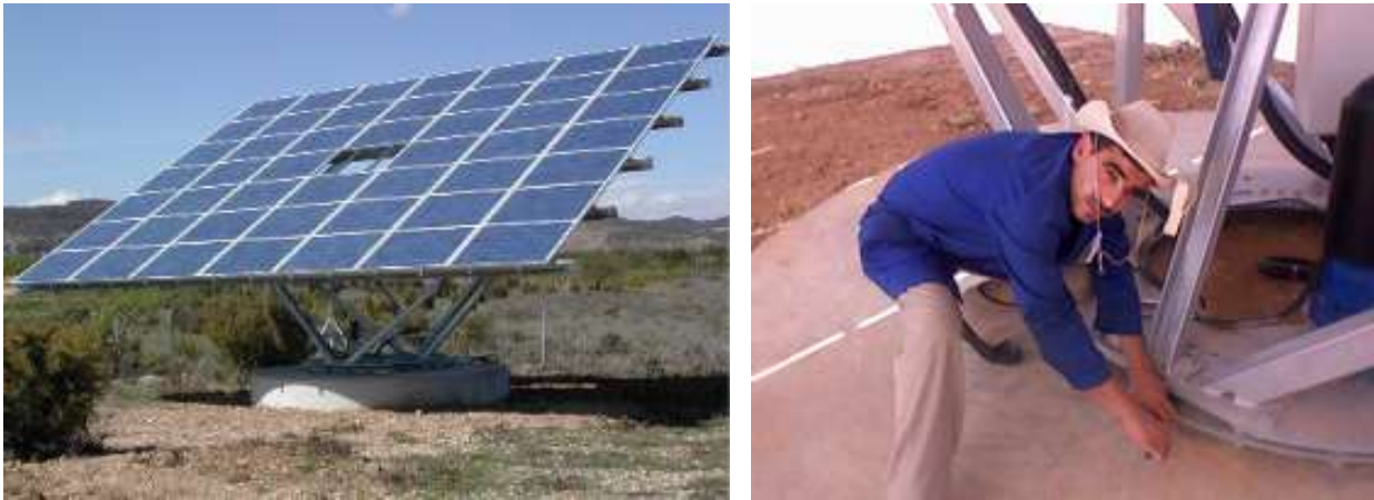
Fig. 1. (Left) dual axis sun tracking Mecasolar MS-2 TRACKER 10+. (Right) Sun tracking MS-2 TRACKER 10+ under installation in Batna, Algeria.
