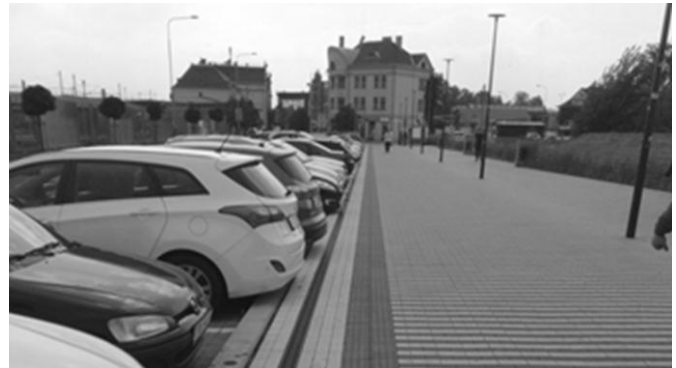
Fig. 10. Unsuitable placement of the artificial guiding line.
