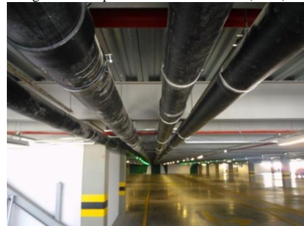
Fig. 3. RHS pipes network. Source: Souza (2013).
