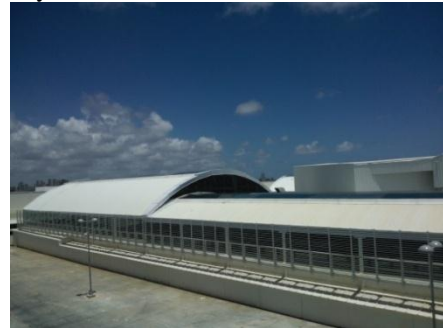
Fig. 2. Rooftop stretch. Source: Souza (2013).
