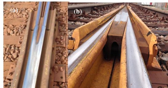
Fig. 5. (a) Conventional frog heel; (b) Low impact heel.
