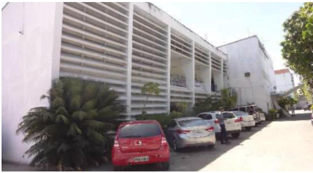
Fig. 2. The building B
